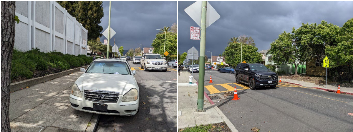
Left: Vehicles were observed parked on the Coolidge Avenue sidewalks.
