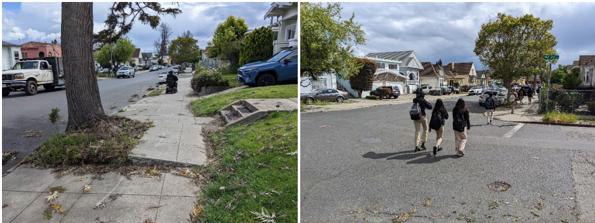
Left: Broken sidewalks present hazards for students and community members.
