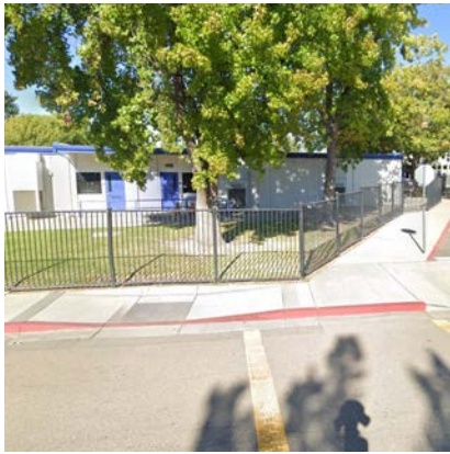
Curb ramp misaligned with the northern end of the crosswalk across Irene Way at Diane Lane.
