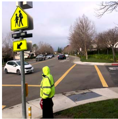
Crossing guard and rectangular rapid flashing beacon (RRFB) at Garaventa Ranch Rd and Hawk St.
