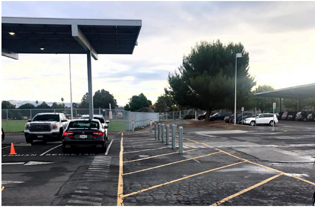
Pedestrian zone in the school parking lot
