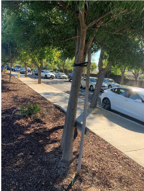
Left: Uneven sidewalk due to root growth from the street tree.
