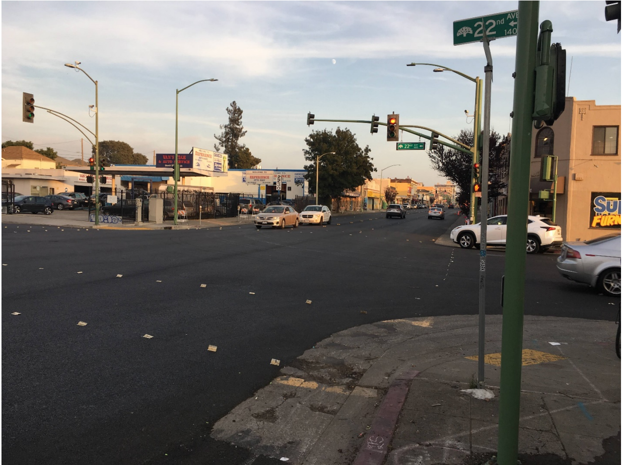
ABOVE: While recently repaved, the intersection of 22 nd Ave and International Blvd does not have striped crosswalks. Large turning radii at corners result in fast-moving turns while students attempt to cross both streets.
