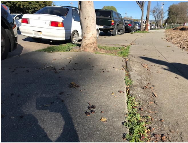
Left: Broken, uneven sidewalk on the south side of Darwin Street.
