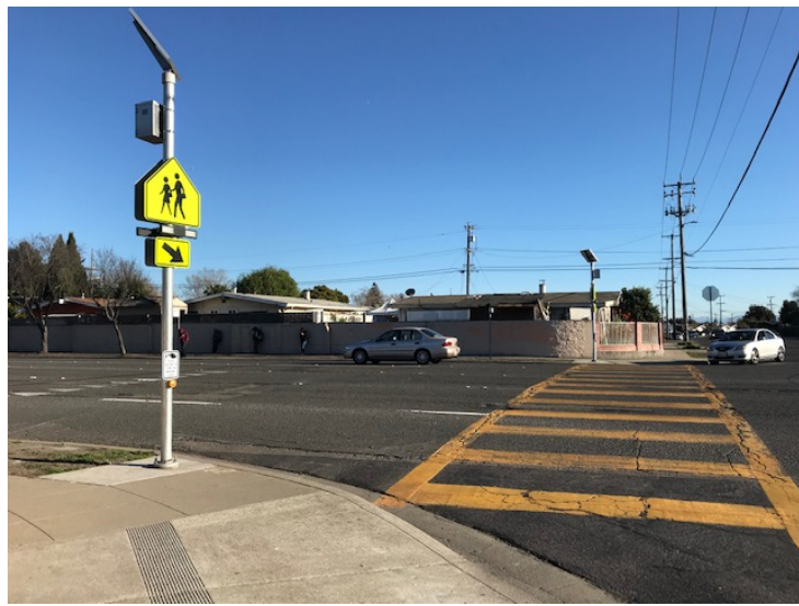
Left: Students wait at the bus stop on Tennyson Road. The bus stop lacks seating and shelter. Right: A high-visibility crosswalk and RRFB across Tennyson Road.
