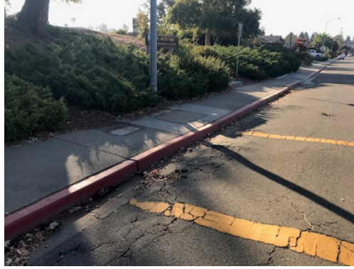
Above: Missing curb ramp and uneven, cracked road conditions on the east side of the north crosswalk.
