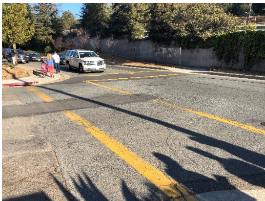
Left: The two transverse crosswalks at the Aliso Avenue/39 th Avenue intersection, looking west. Right: Looking down 39 th Avenue, towards the drop off loop. The advance stop markings are very faded at the approach.
